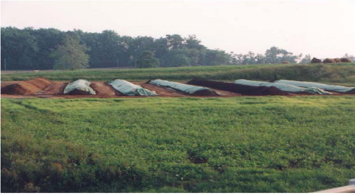
A Composting operation showing a soil cement pad and grass buffer for run-off control
